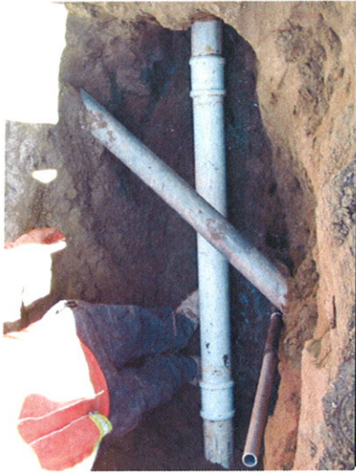
DAMAGED PIPE REMOVED AND REPLACED
