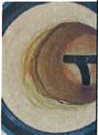
COMPLETED APPLICATION ON MANHOLE SHAFT & BASE
