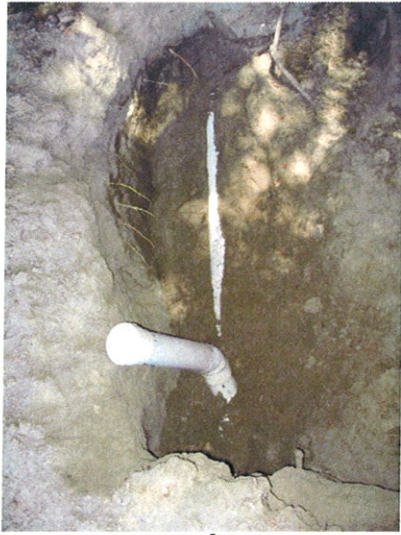
DAMAGED PIPE REMOVED AND REPLACED
