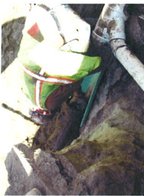
Defective orangeburg mainline sewer pipe was removed from the Sage Street Alley and replaced with plastic PVC pipe
