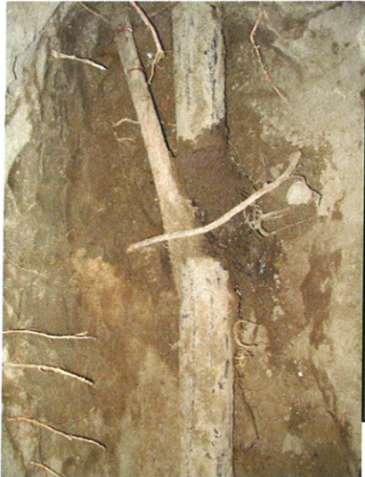
ROOT INTRUSION IN VSD LATERAL
