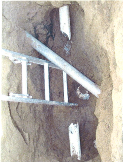
DAMAGE TO VSD LATERAL BY UTILITY CONTRACTOR
