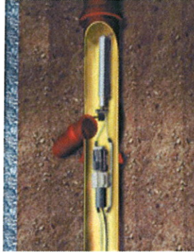
Service laterals are restored internally with robotically controlled cutting devices
