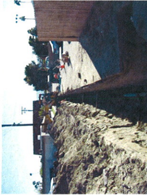
Defective orangeburg mainline sewer pipe was removed from the Deglet Noor Alley and replaced with plastic PVC pipe.
