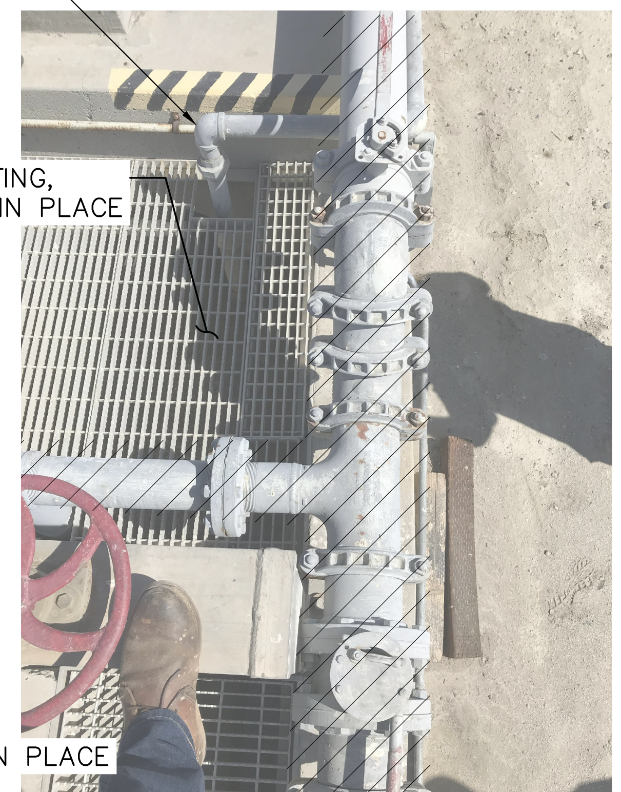
PHOTO EXISTING PIPING TO BE DEMOLISHED (B)
