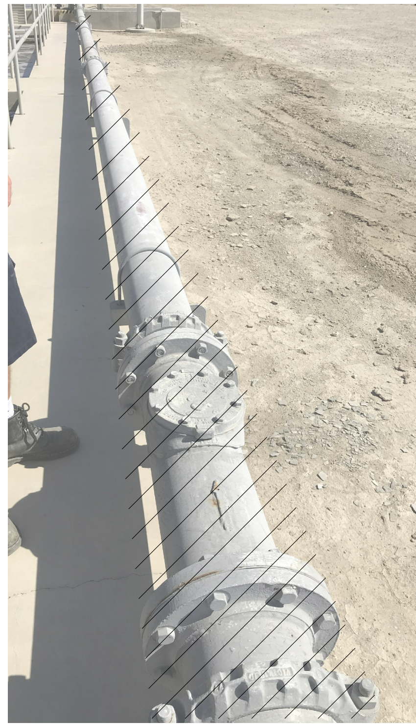
PHOTO EXISTING FLOWMETER TO BE DEMOLISHED (F)
