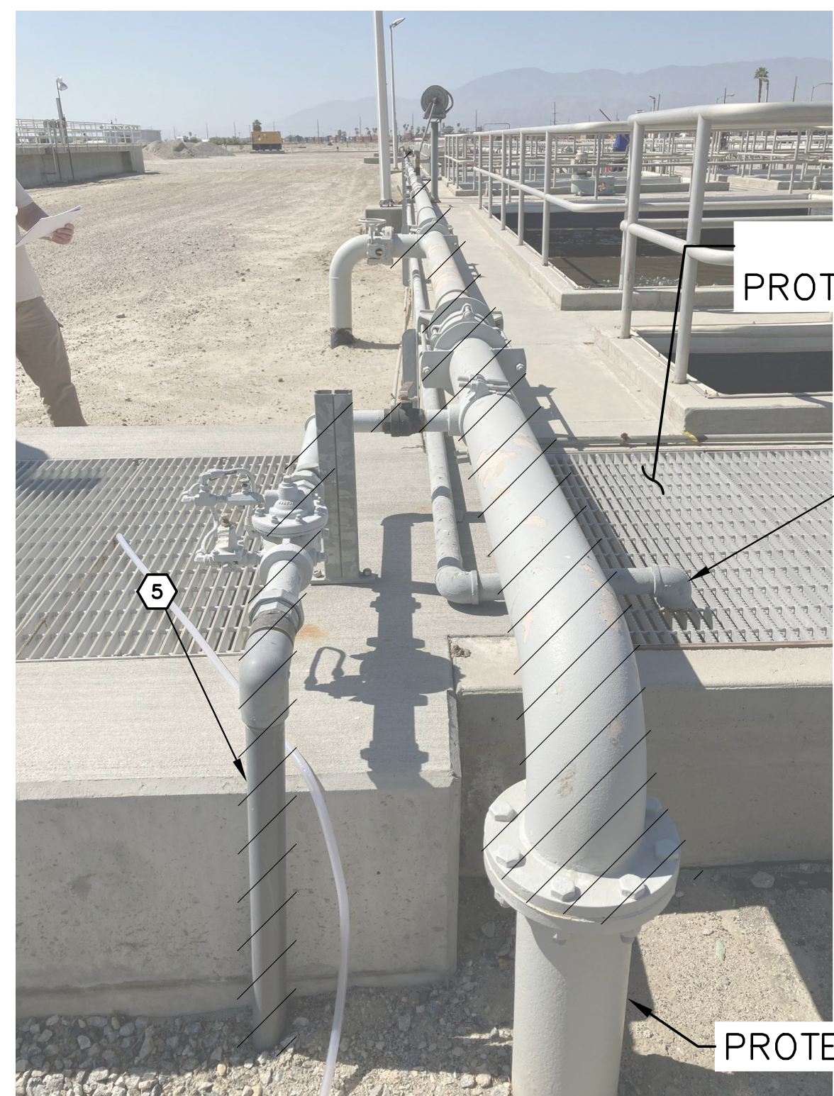
PHOTO PROJECT START LOCATION (A)
