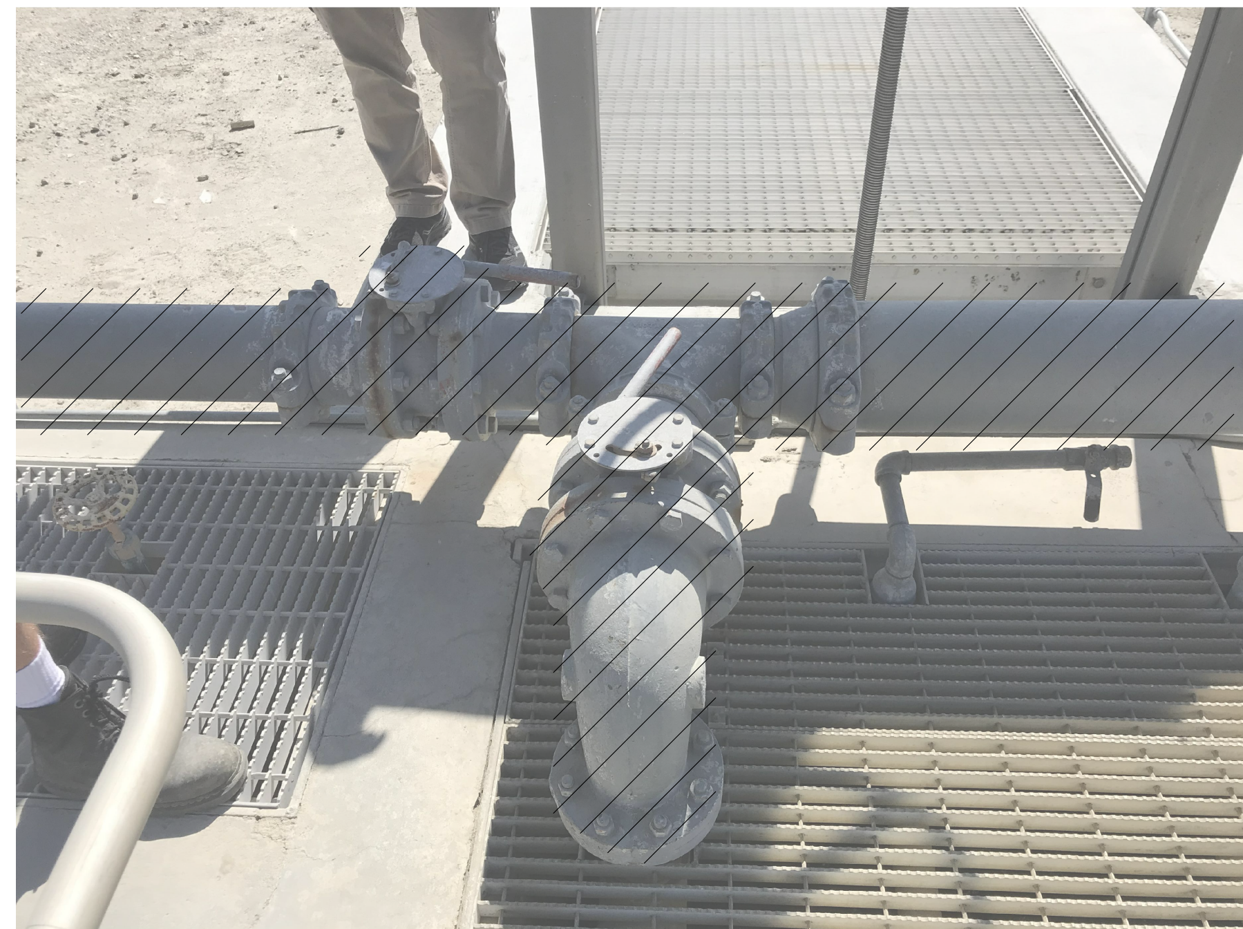
PHOTO EXISTING PIPING TO BE DEMOLISHED D
