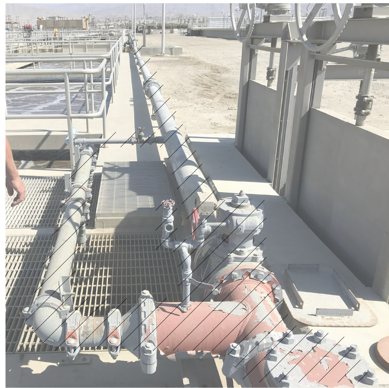
PHOTO EXISTING PIPING TO BE DEMOLISHED (H)
