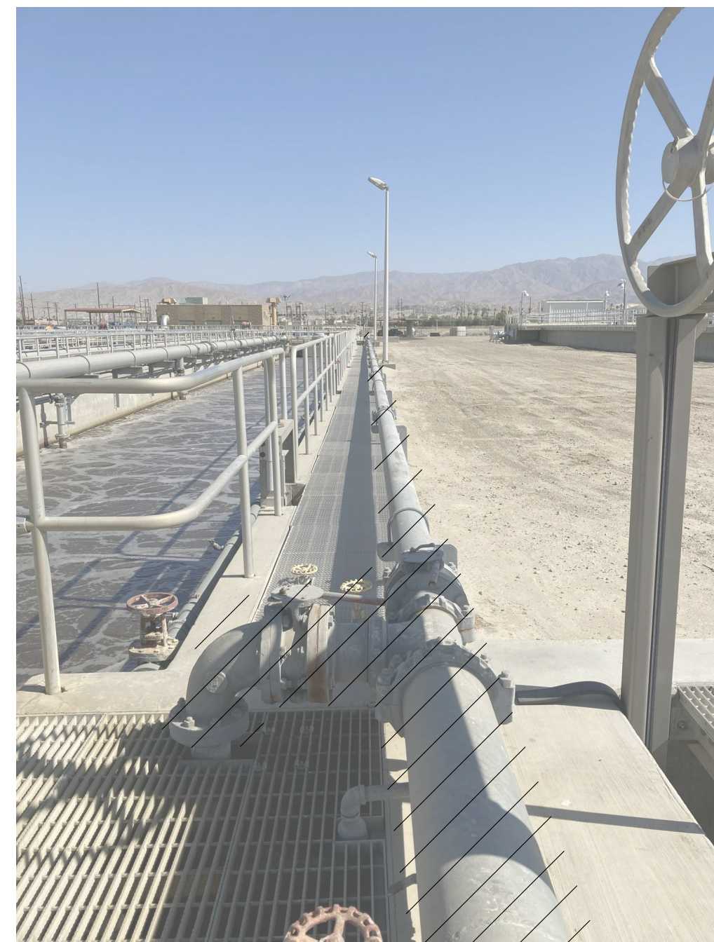
PHOTO EXISTING PIPING TO BE DEMOLISHED E
