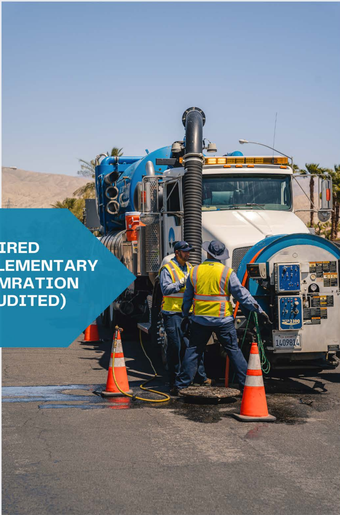
Sanitary Collections Crew Jetting Sewer Lines
