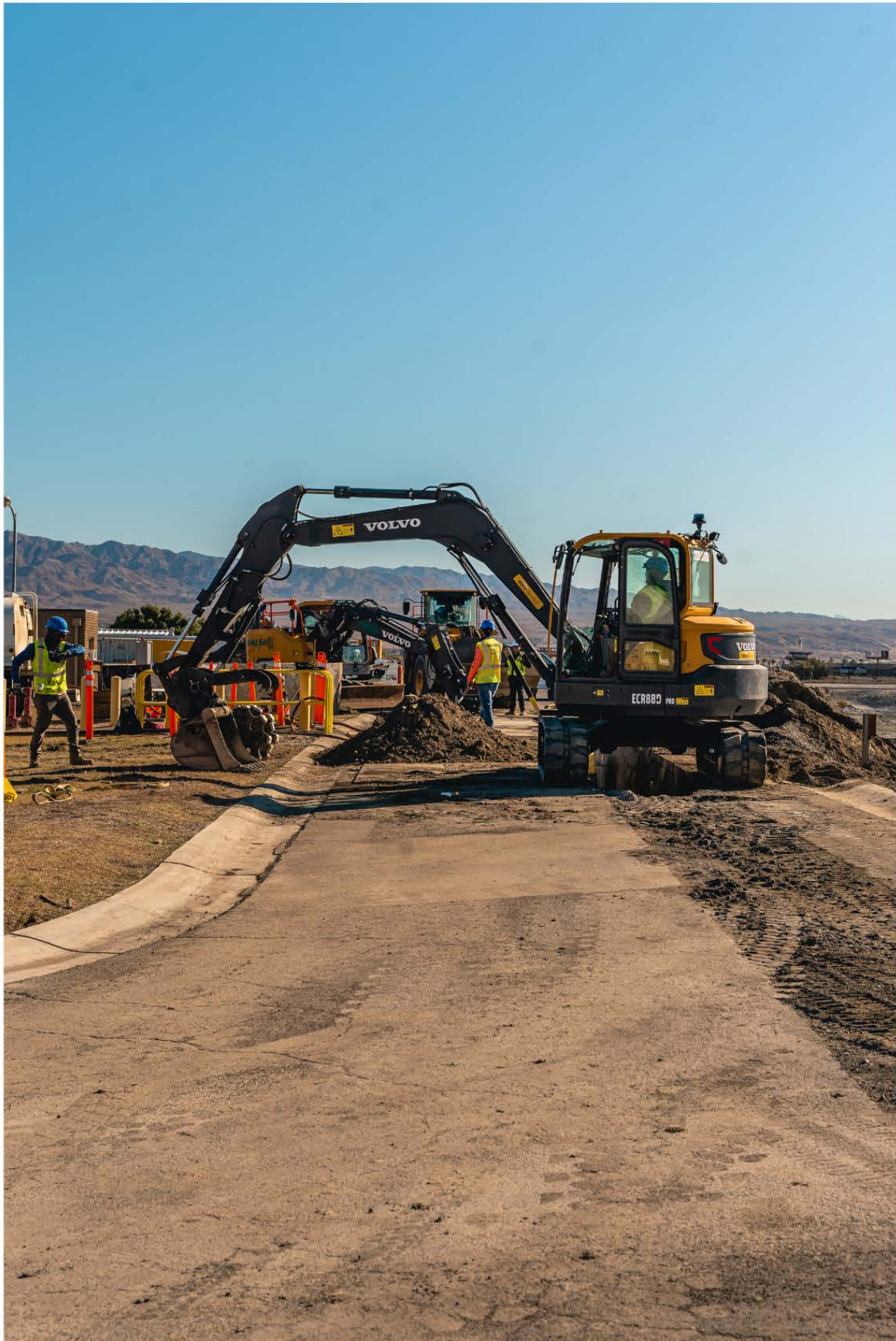
Recycled Water Project - Phase I Piping Installation
