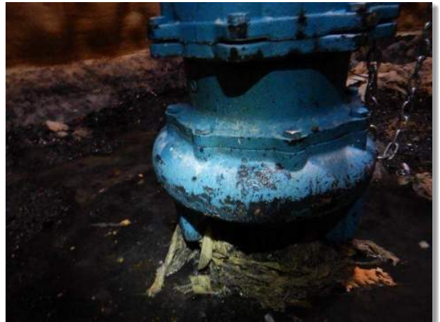
Photo 3-52. Pump base in good condition, typical
