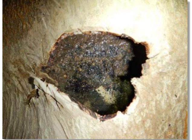
Photo 3-38. Close-up of concrete behind liner
