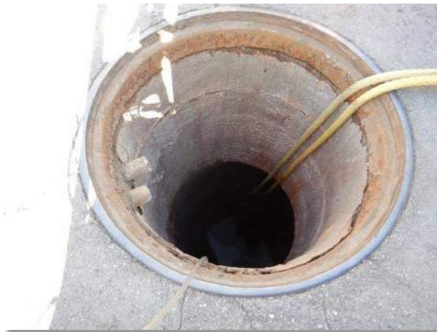
Photo 3-71. Wet well framing
