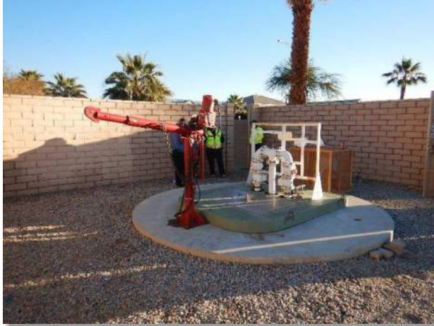
Photo 3-31. Wet well exterior
