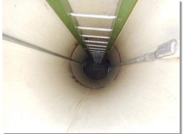
Photo 3-6. Dry well interior, topside
