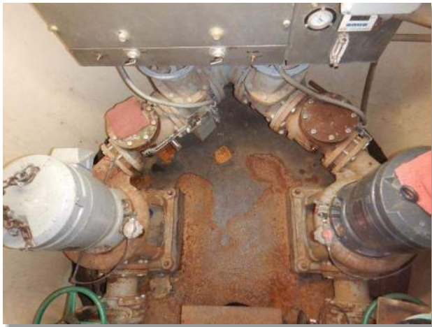
Photo 3-59. Dry well Interior
