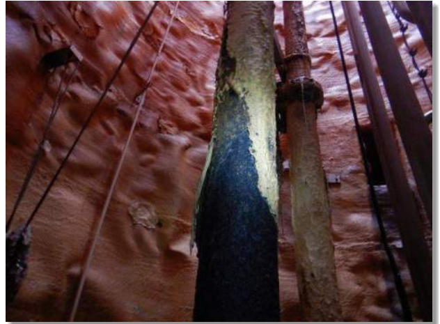
Photo 3-44. Epoxy coating begins at 6-ft from floor
