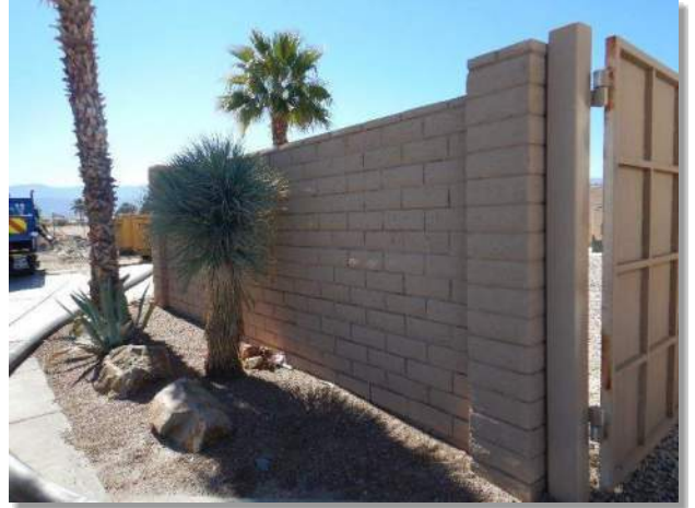
Photo 3-24. CMU perimeter wall
