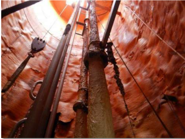
Photo 3-43. Epoxy coating on pump discharge piping above 6-ft
