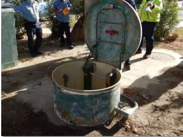
Photo 3-5. Dry well access hatch exterior
