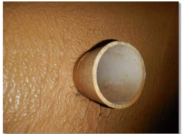
Photo 3-84. 4-in PVC lateral
