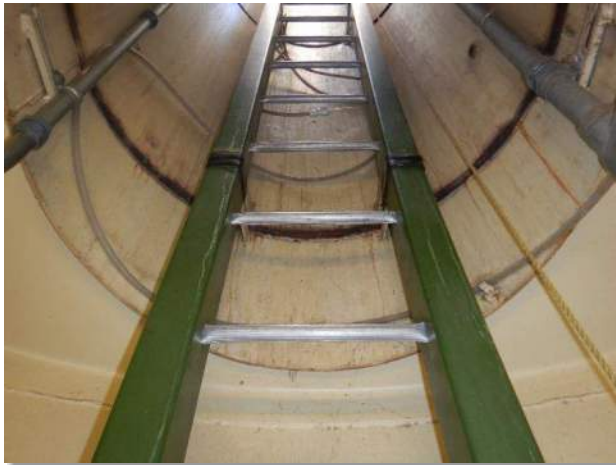
Photo 3-7. Dry well interior walls and access ladder
