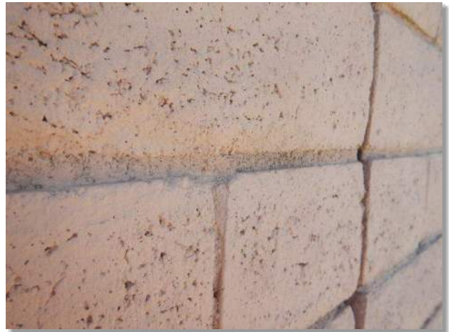
Photo 3-26. CMU mortar pointing in good condition
