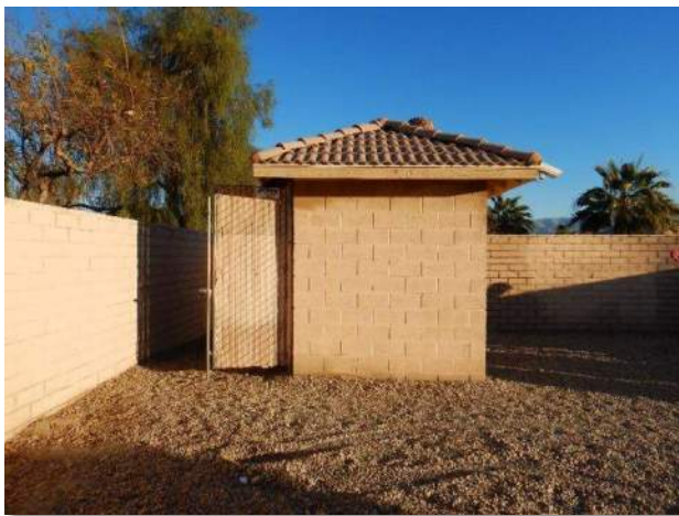
Photo 3-27. Electrical building exterior
