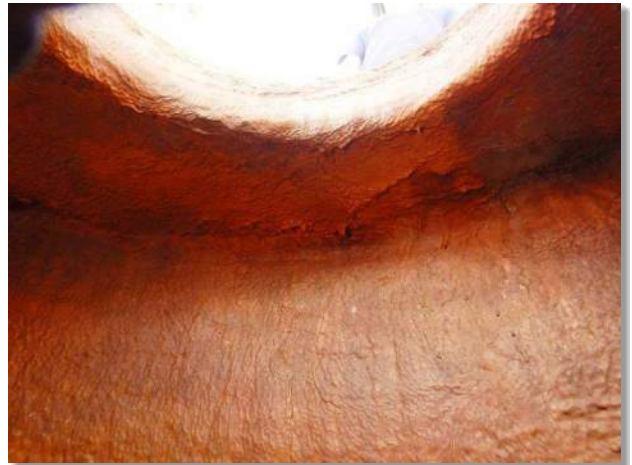
Photo 3-18. Wet well interior, epoxy liner at ceiling
