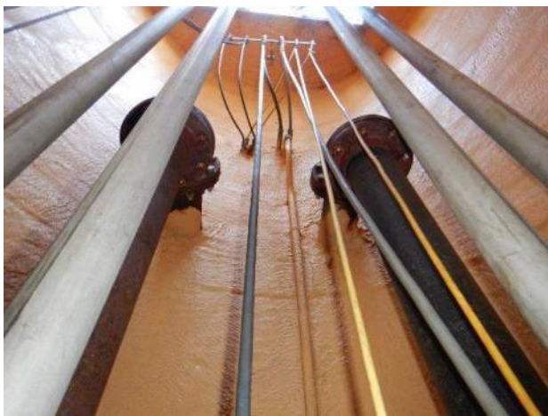
Photo 3-89. SST guide rails in good overall condition
