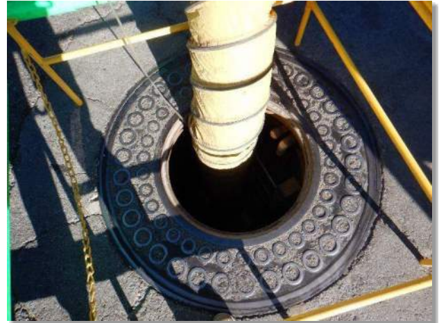
Photo 3-54. Dry well exterior framing
