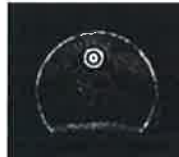
SIPHON WITH SIGNIFICANT DEBRIS
