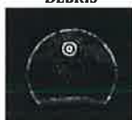
SIPHON WITH SIGNIFICANT DEBRIS
