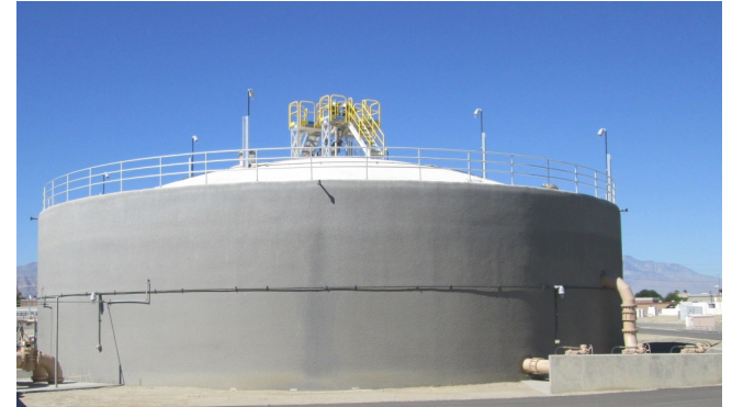
Existing Digester No.2
