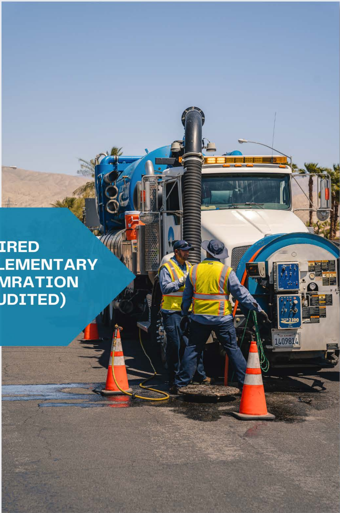
Sanitary Collections Crew Jetting Sewer Lines
