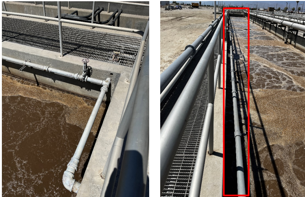
Figure 1: Piping to be Replaced as part of this Project
