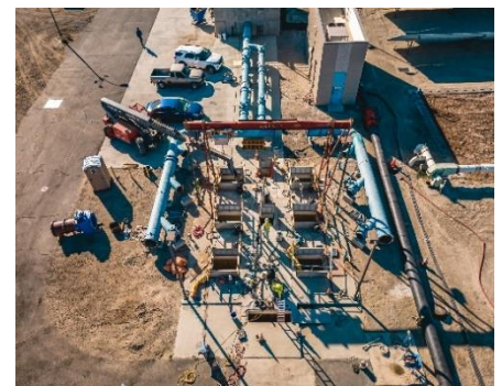
Influent Pump Station Rehab
