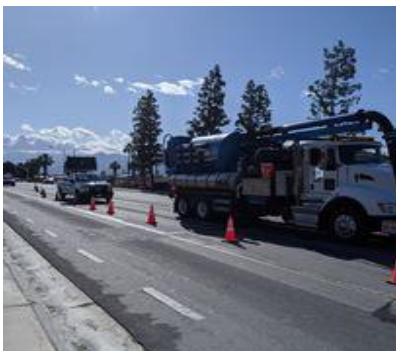
Collection System Rehab – Phase I
