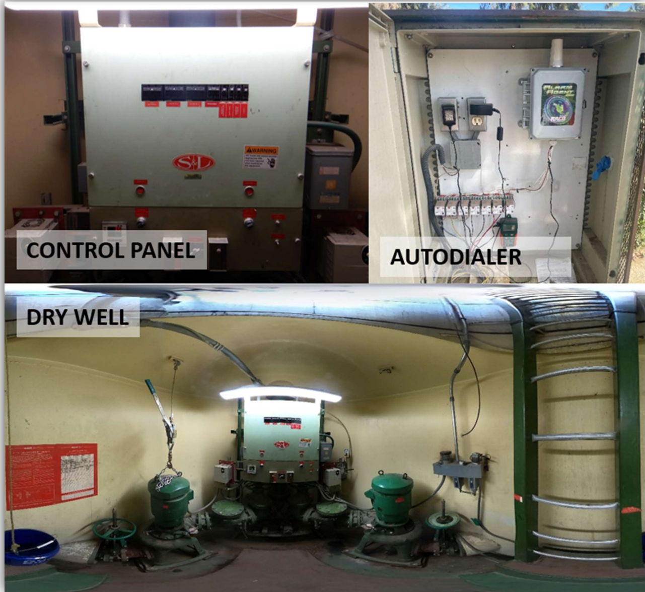
FIGURE 5: Barrymore Lift Station Photos
