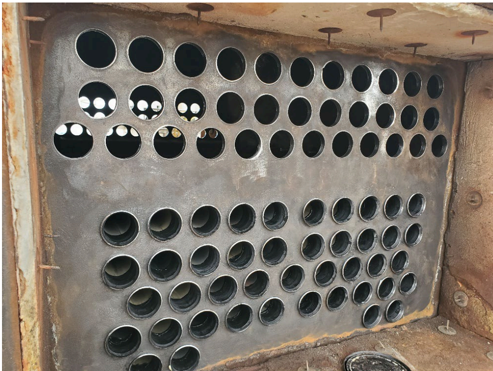
Replaced Heat Transfer Tubes
