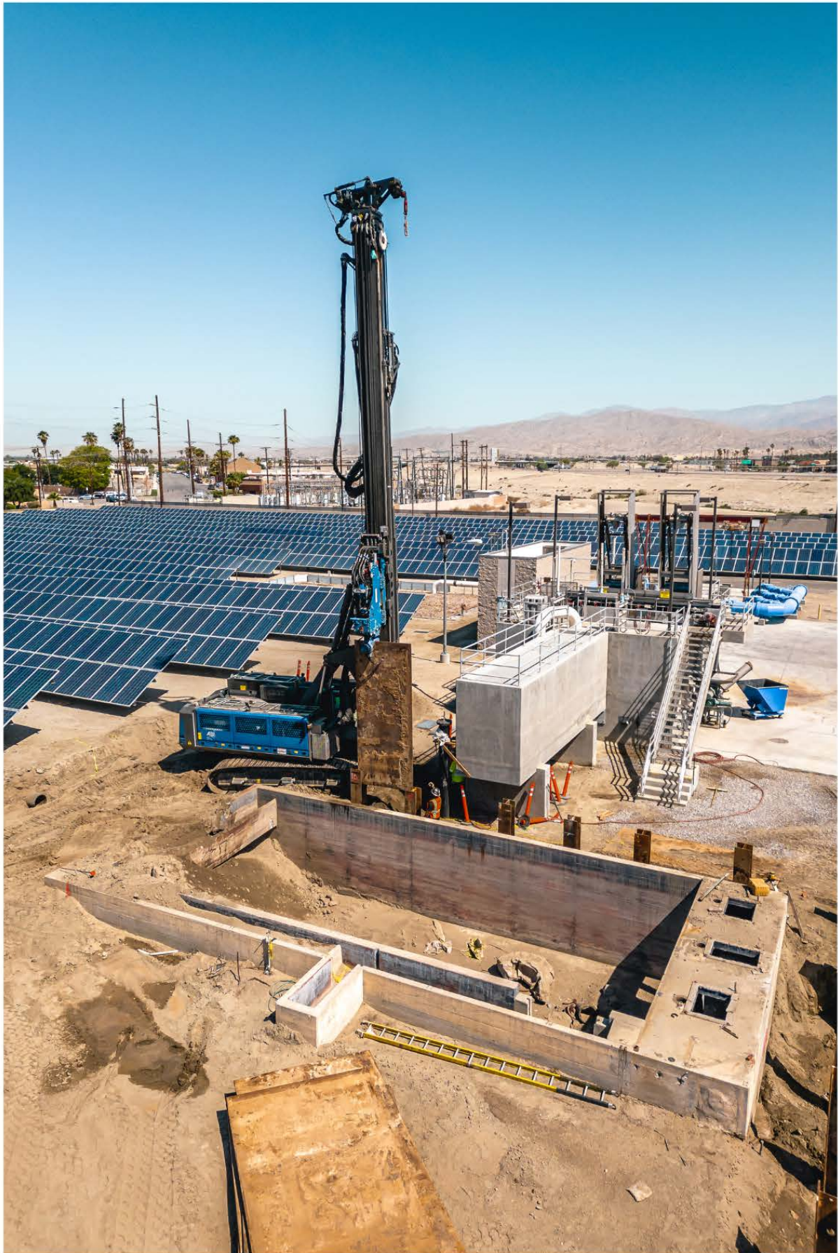
Demolition of Old Contact Chamber
