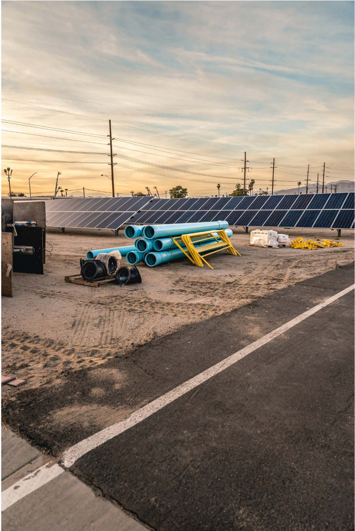
Wastewater Facility Recycled Water Project Sewer Piping
