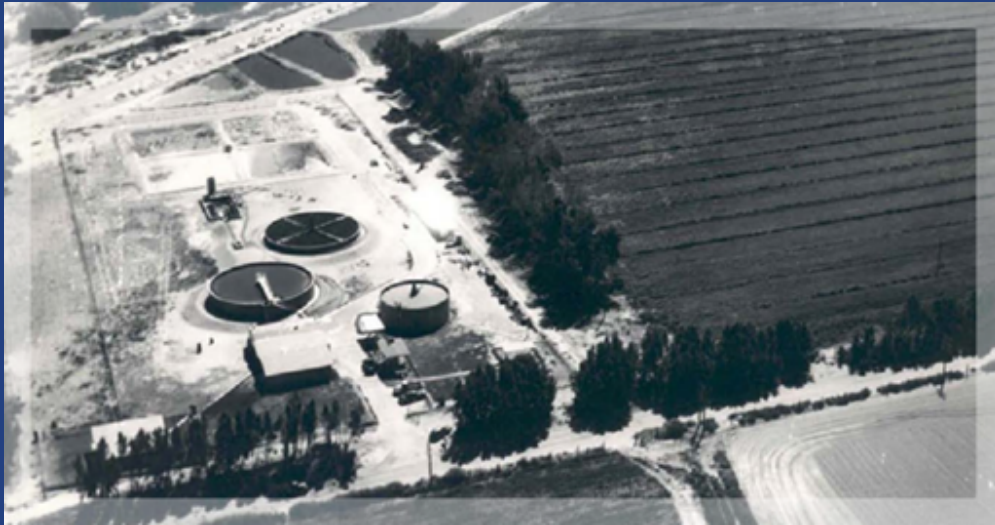
1950's VSD Treatment Plant
