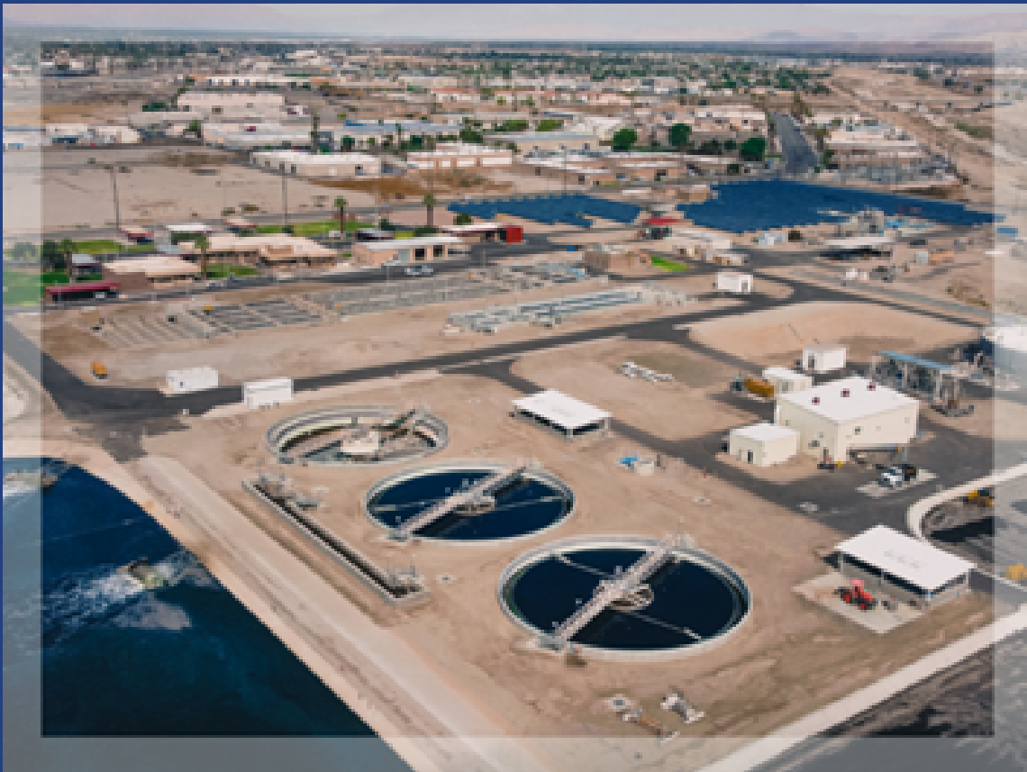
Overview of Valley Sanitary District
