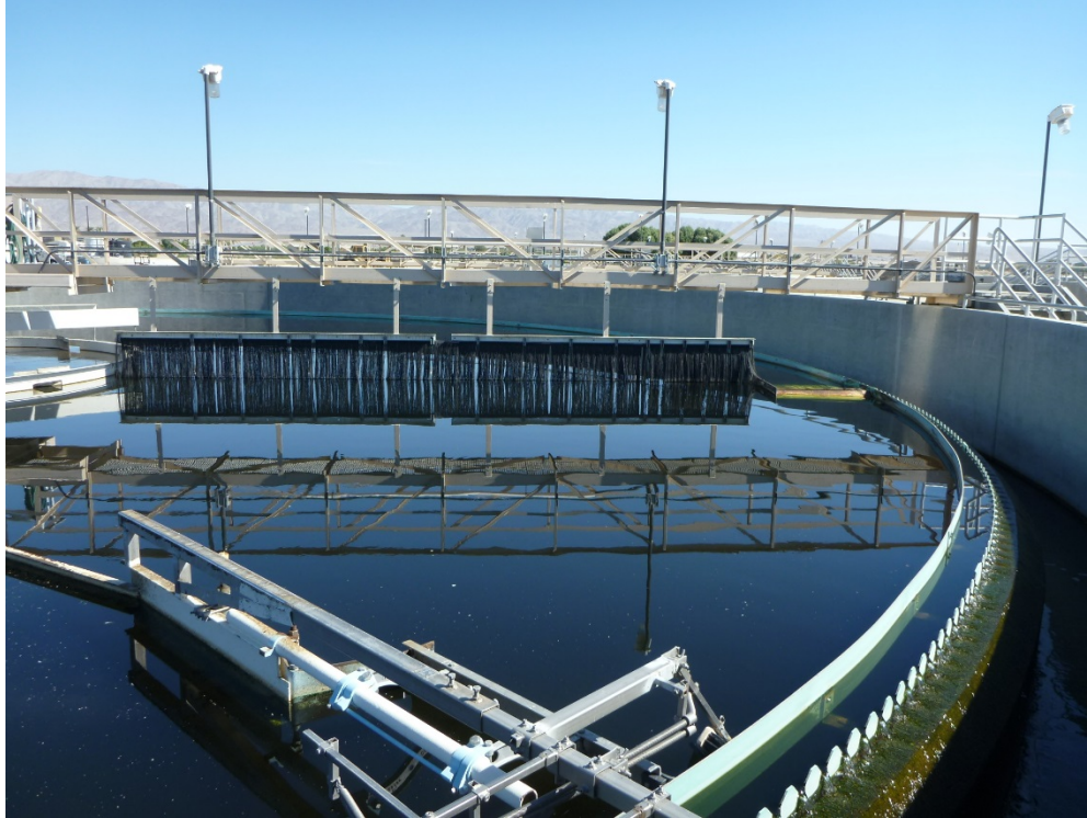
Figure 3-7 Secondary Clarifier
