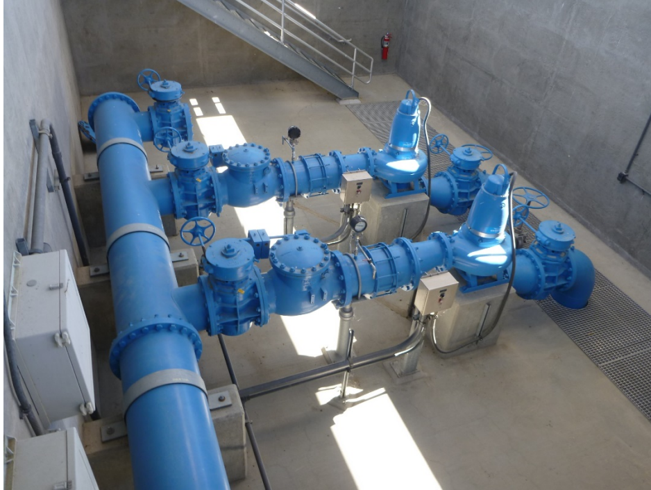
Figure 3-6 Clarifier No. 3 RAS Pumps
