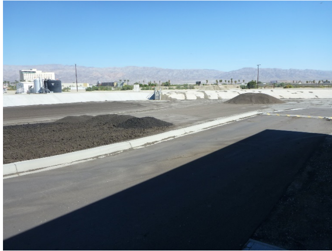
Figure 3-15 Sludge Drying Bed
