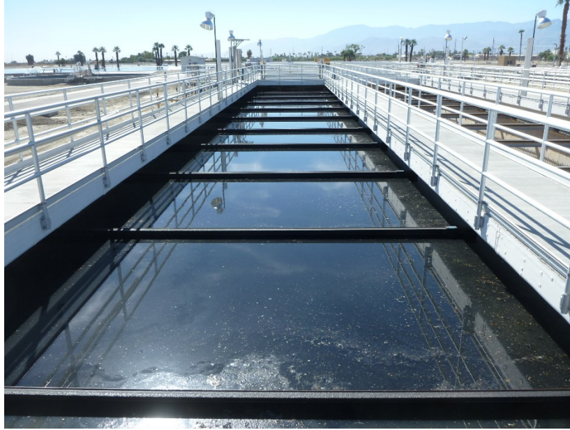
Figure 3-4 Primary Clarifier
